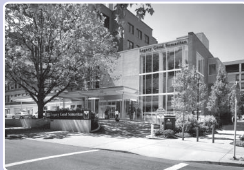
Legacy Good Samaritan Hospital & Medical Center
